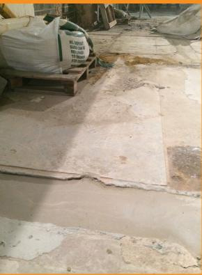
Channels were backfilled and level differences ramped down.
