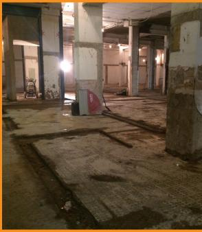
Level differences and channels in the existing floor called for a high level of preparation.
