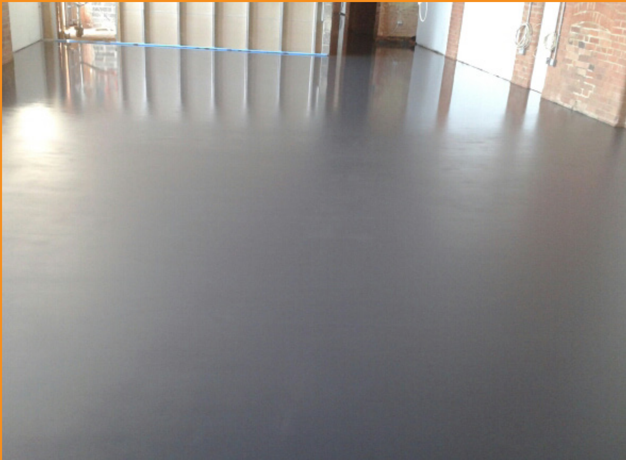
Screed to Main Exhibition Area
