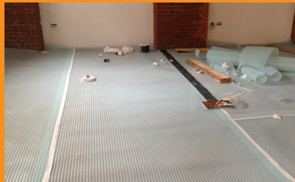
DPM being applied
