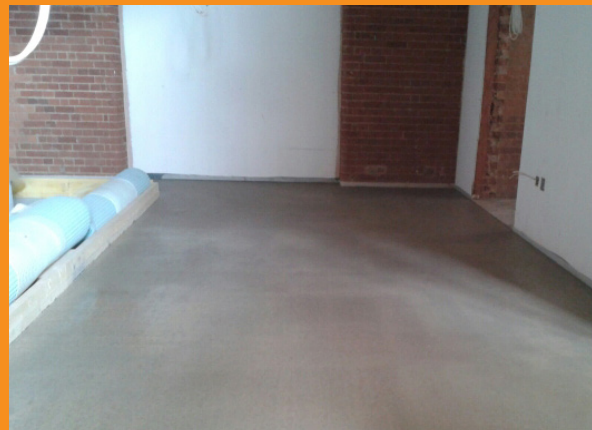
Screed in curing process in the Throne Room
