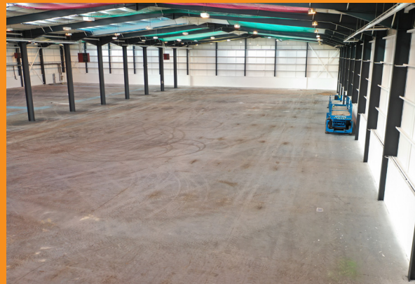
Above: Internal unit space refurbishment stages
