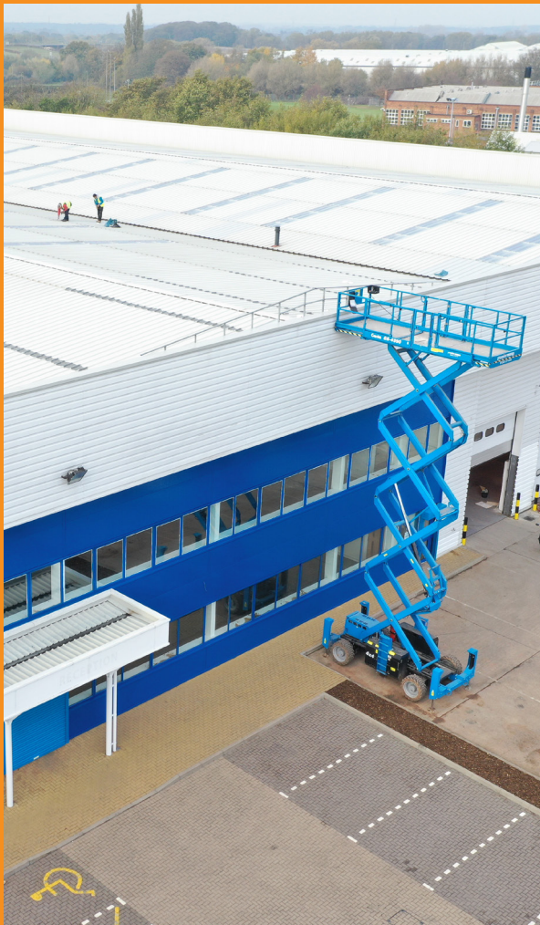
Below: External roof repairs
